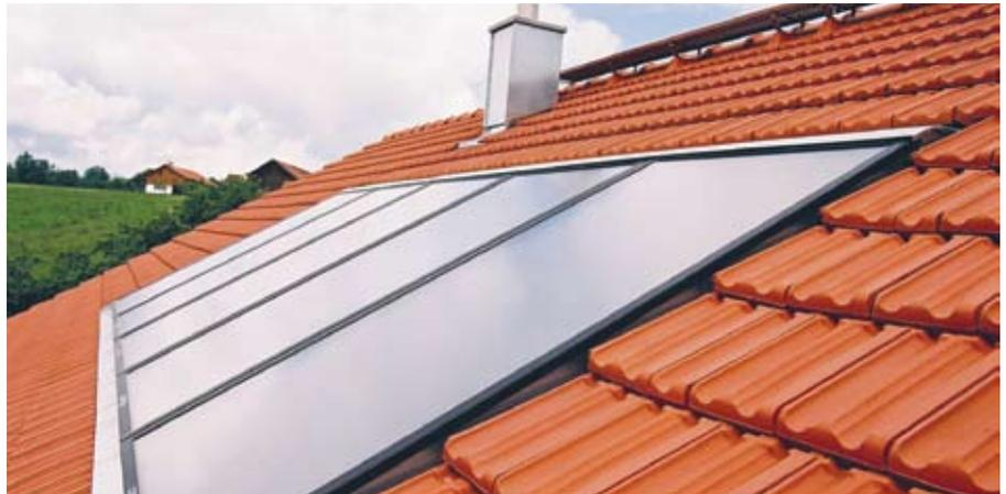
Roof-integrated flat-plate solar thermal collectors.
