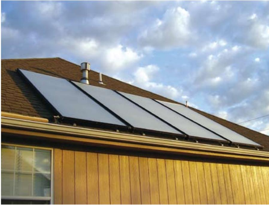
*A residential solar hot water system using four Heliodyne GOBI collectors.*
