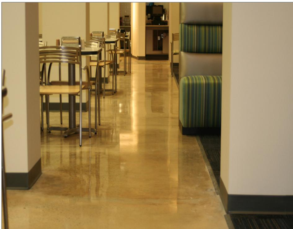
Chemical densifiers used in polished concrete flooring seal off any pores that water or contaminants can penetrate giving a sanitary surface.
