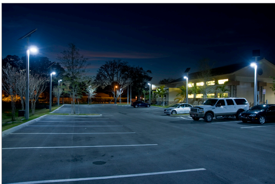
Solar-powered LED street lights illuminate a parking lot in Parkland, FL.
