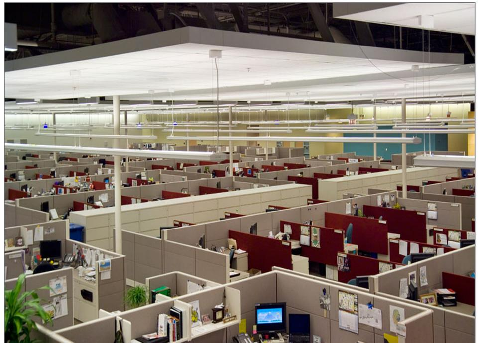
Energie Lighting direct indirect lighting system incorporated reflective Miro Aluminum to direct light where needed providing better color rendering and visual comfort for facility occupants at BlueCross call centre.
